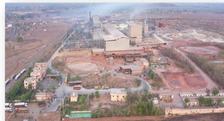
Rajoua Plant in Sagar
